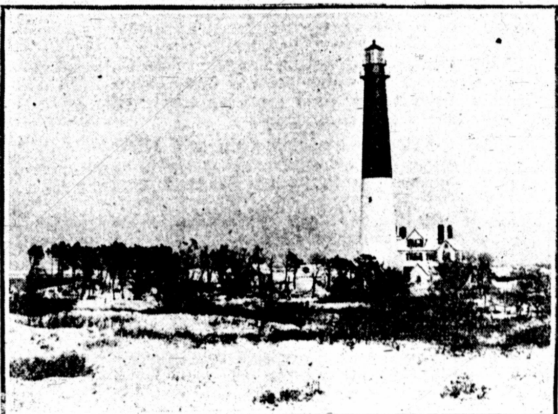
The U. S. Bureau concerning such things has ruled that Barnegat, the oldest lighthouse on the Atlantic coast, is no longer safe and must go, its foundations having been undermined by the sea.
