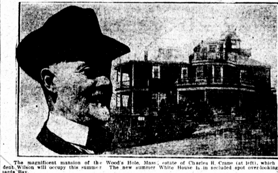
The magnificent mansion of the Wood's Hole, Mass., estate of Charles R. Crane (at left), which President Wilson will occupy this summer. The new summer White House is in secluded spot overlooking Buzzards Bay.
