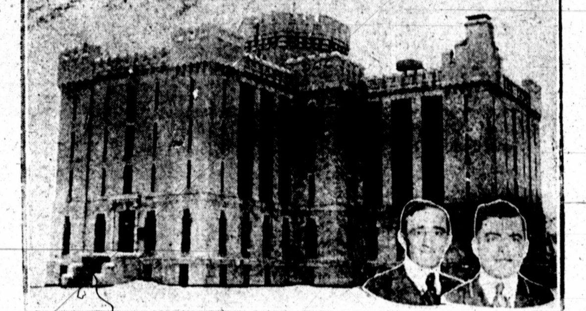
If the house situation in Hackensack, N. J., is not relieved by May 1st city officials are seriously considering throwing open the jail to provide living quarters for some of the homeless families. Insert: Warden John B. Storrs and Sheriff Joseph Kinzley, Jr., who will probably play landlord to the homeless Hackensackers.
