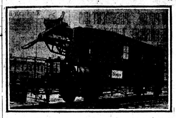
German scientists have discovered a new use for airplane propellers. During recent tests held in Berlin, a railroad engine equipped with sirplane propellers and engines at both ends covered a distance of 300 kilometers between Berlin and Hamburg in one hour. The motors are of 160 horse-power. It is believed that the propellerdriven engines will effect a tremendous saving in coal, which essential is sadly lacking in Germany.
