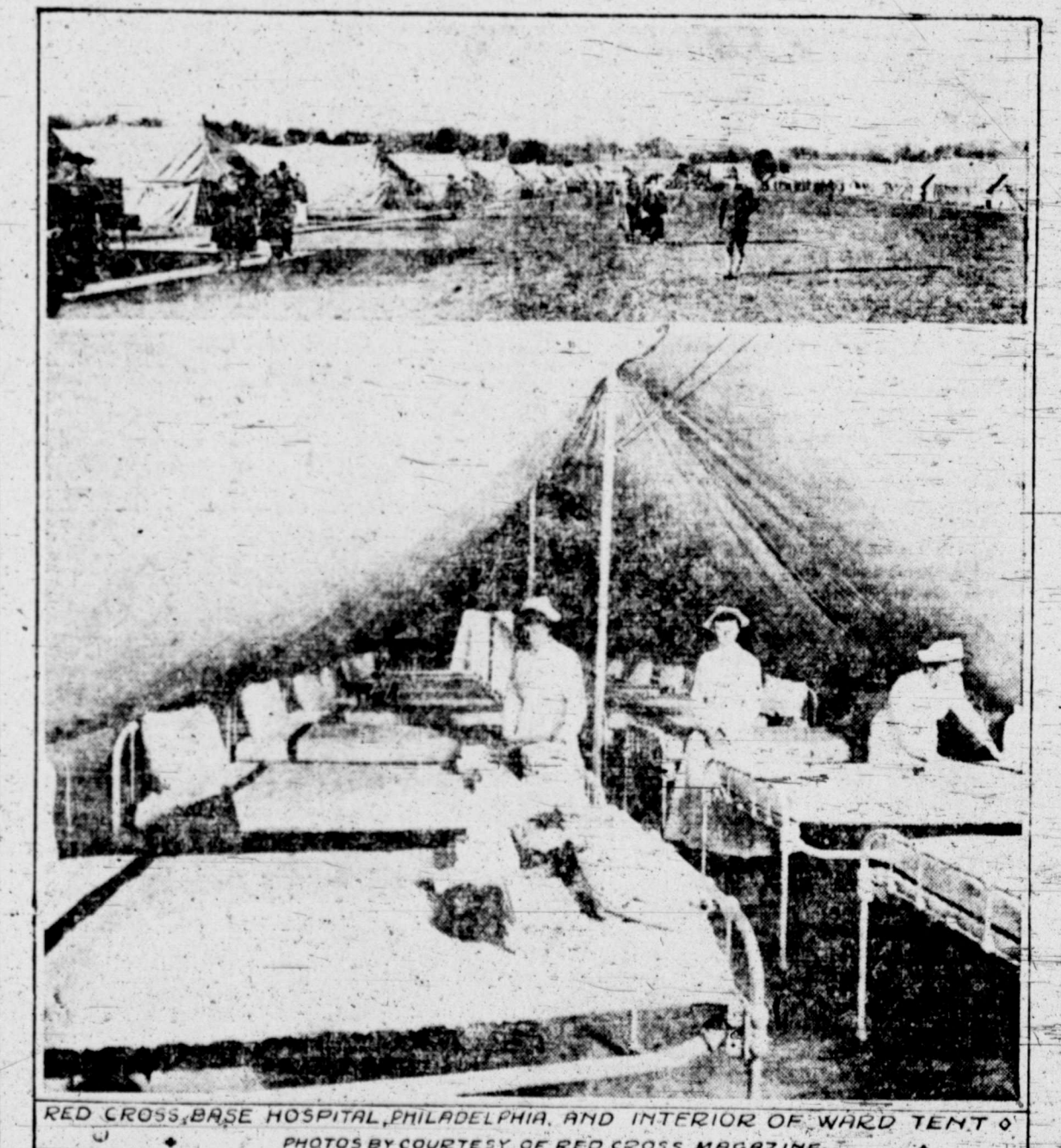
RED CROSS BASE HOSPITAL, PHILADELPHIA, AND INTERIOR OF WARD TENT
