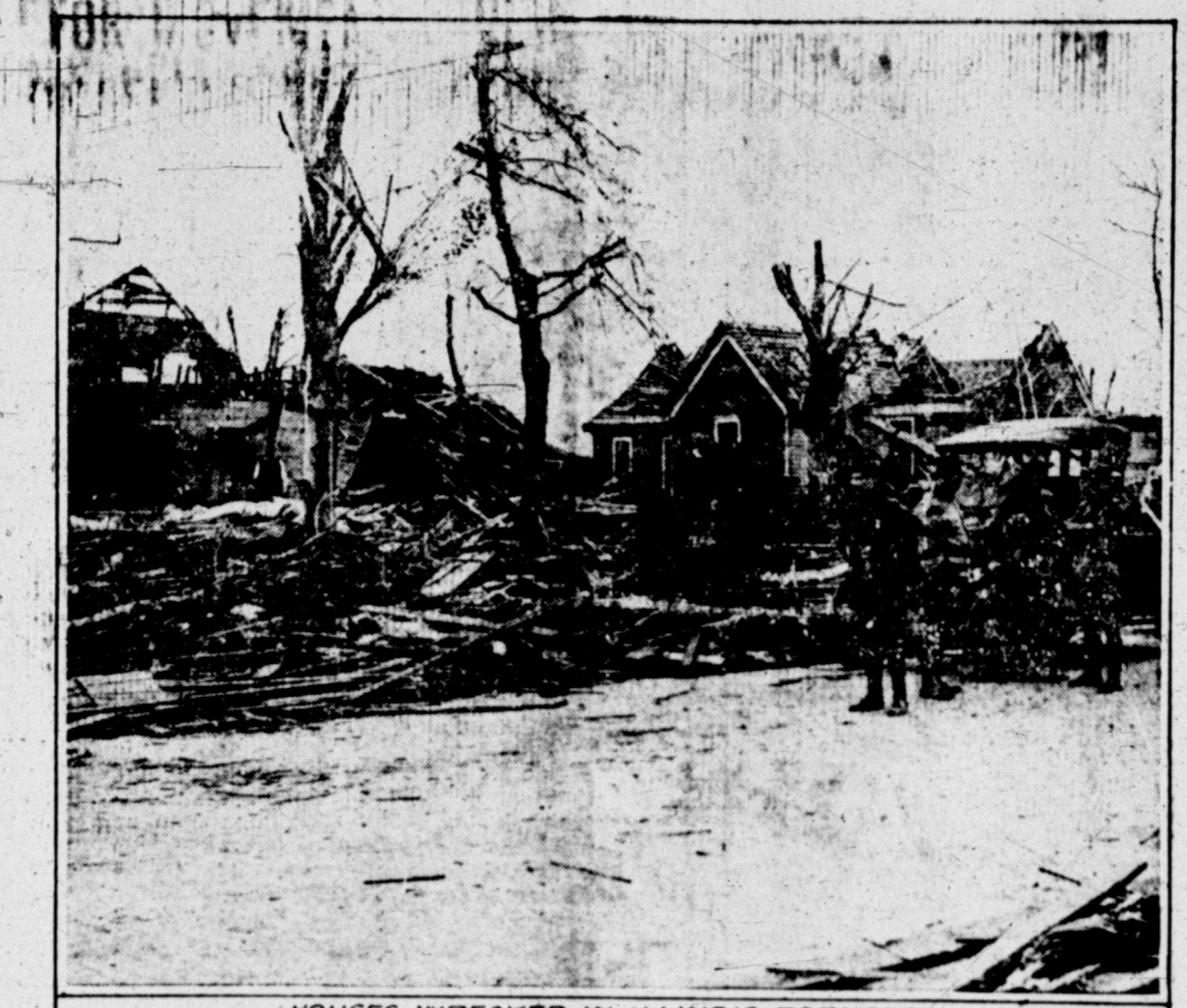
HOUSES WRECKED IN ILLINOIS TORNADO
