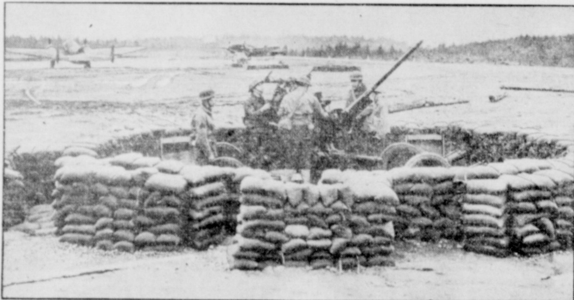
Revetments augmented by mobile and stationary anti-aircraft emplacements, are part of the defenses in the Pacific northwest coastal area. On the alert, a gun crew mans a 37-mm. anti-aircraft piece. Planes in the background would be in the air at once in case of alarm.
