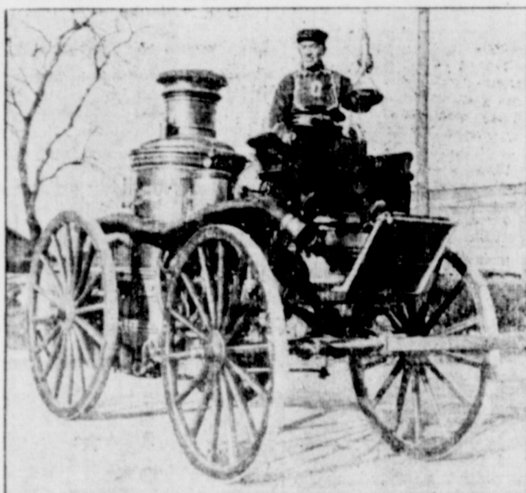
FIGHTS FIRE WITH FIRE—Veteran of many battles with flames, Thomas C. Durant, first steam fire engine west of the Missouri river, will engage in a new battle when it is scrapped for precious metals. Thomas Kenworthy, 65, of Omaha, is the last remaining old-timer who was engineer for the old Durant. Engine will yield 700 pounds of brass, 100 pounds of copper, and 4800 pounds of steel.
