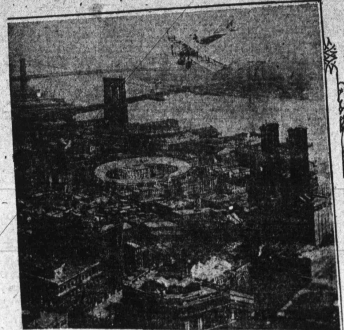
The circular landing track could be carried on stilts above several buildings, without cutting off light or air.
