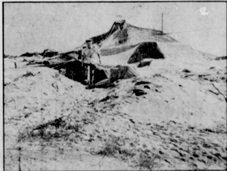
Cleverly camouflaged desert headquarters tent has been dug into the sand on either side of a truck. From the air, this structure on the western desert looks like just another sand dune.
