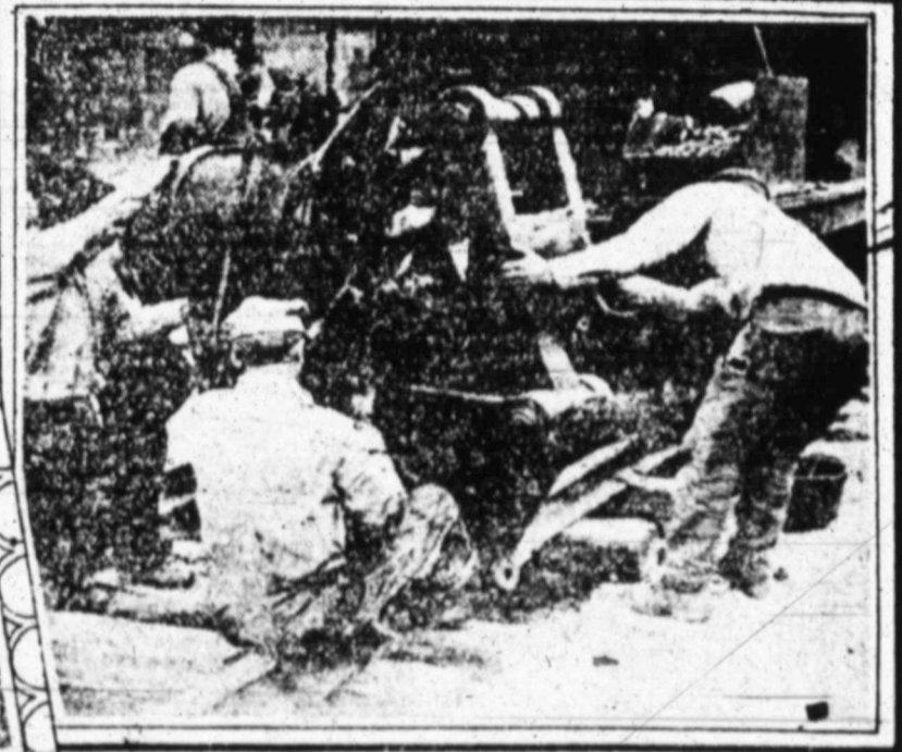
AUTOMATIC RIVETER, OPERATING UNDER A PRESSURE OF 80 TONS COMPRESSED AIR
