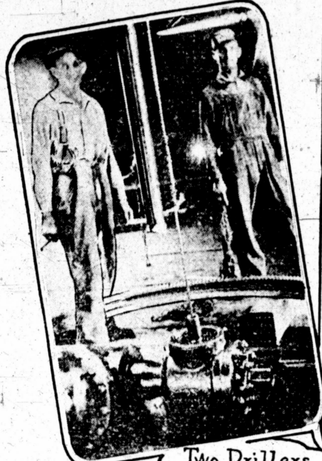
Two Drillers at ARNOLD No. 1
