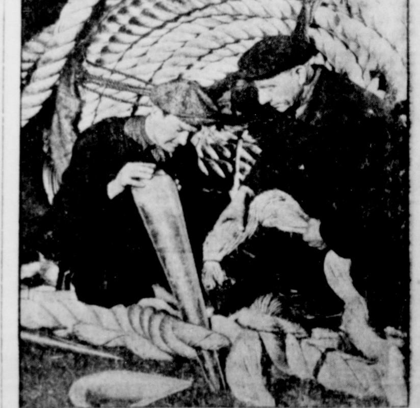
Canada is playing a major role in overhauling and repairing naval and cargo ships of the United Nations. Here workmen splice heavy hawser in the sail loft of a naval yard.
