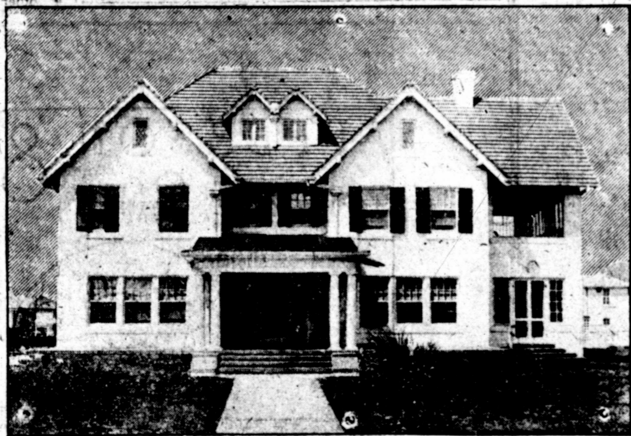
Home of Mr. J. W. Evans, Houston, Texas. Designed and Erected by The Russell Brown Company. HOUSTON, WICHITA FALLS, DALLAS
