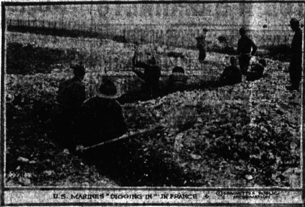
"Digging in" in France, training for modern warfare, consists mostly in digging one trench after another, and the United States marines, realizing the importance of this training, go to it with a will.
