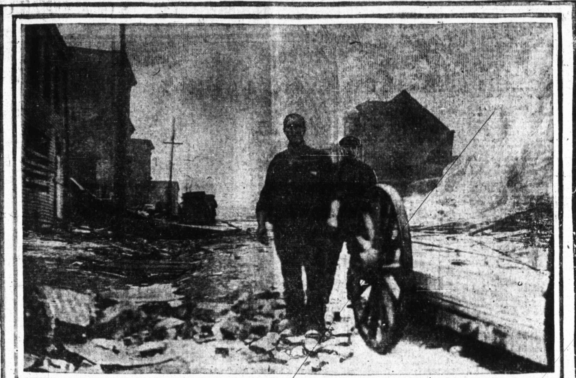
BARRINGTON STREET AFTER EXPLOSION
