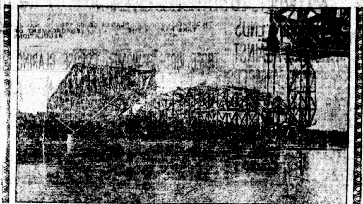
One year after the fatal accident at Quebec. The span is 122 feet above the big Quebec bridge another attempt the St. Lawrence river. It is 640 feet to raise into place the center span and was brought down the river that fell was made, and it was suspended to the bridge site on pontoons. It was suspended from the opposite ends of the bridge by chains and raised into place by powerful jacks.
