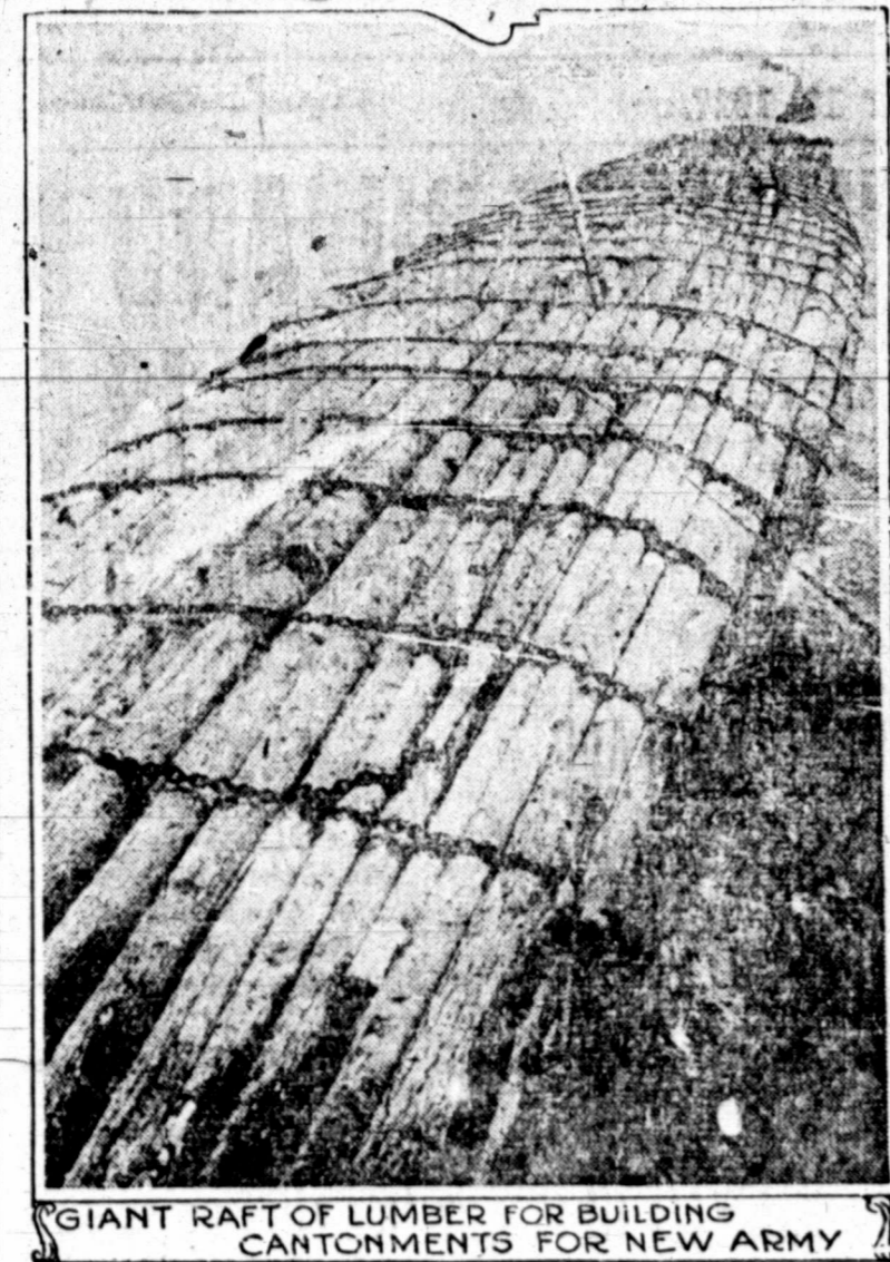
GIANT RAFT OF LUMBER FOR BUILDING CAMPMENTS FOR NEW ARMY
