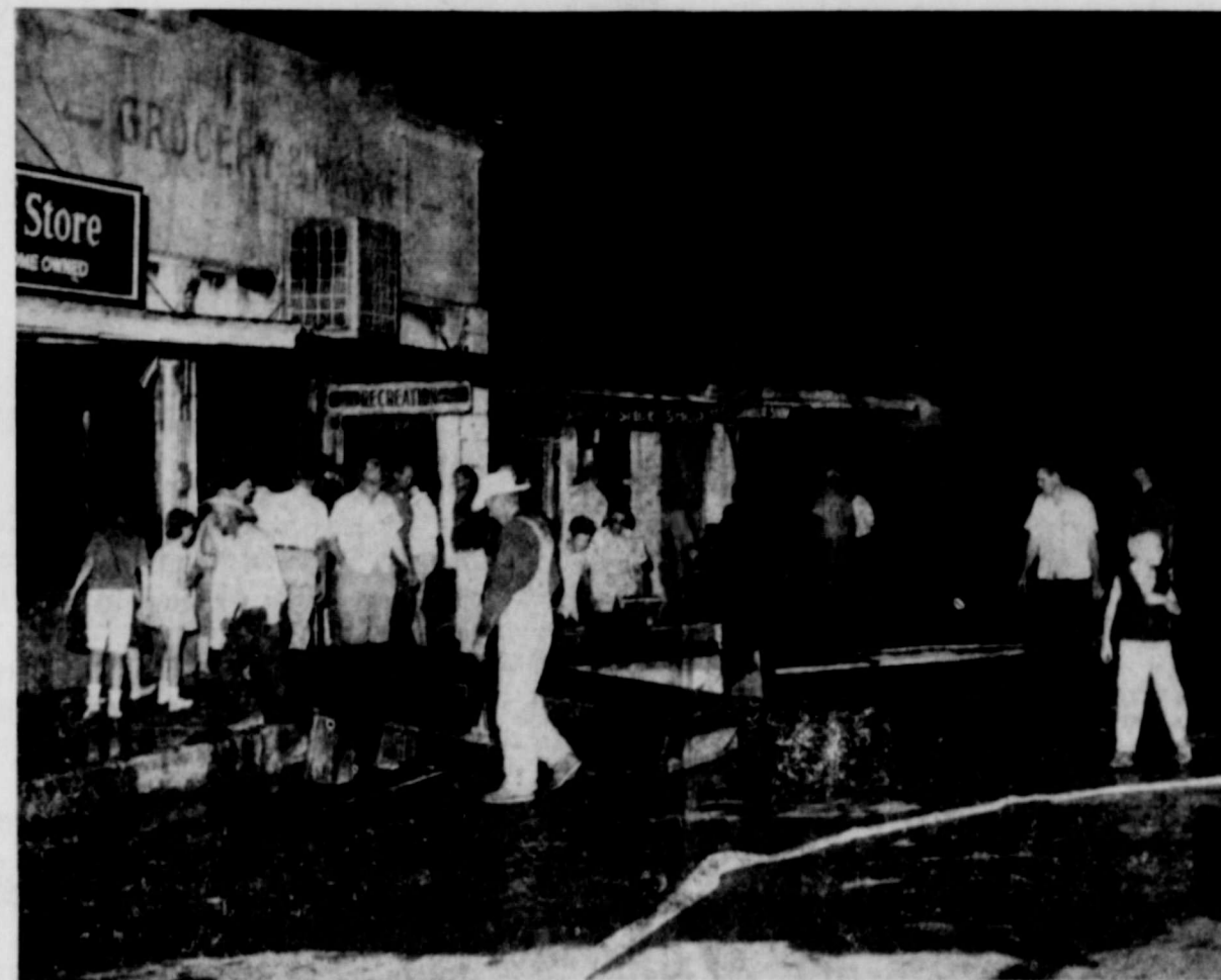
FIRE RUINS—Ruins of three of the four businesses in Tuesday's fire are shown here. At left is Hico Recreation Center,
