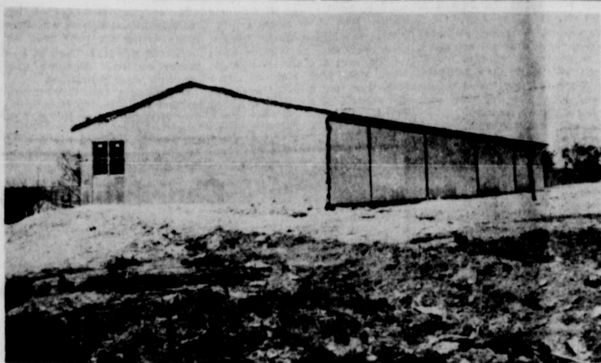
NEW BUS FACILITIES—Shown here is the recently completed school bus storage facilities. The building, erected west of the high school plant, is 36x100 feet, and contains seven bus stalls plus two other stalls for shop space. Built of sheet iron construction, the building is completely enclosed.
