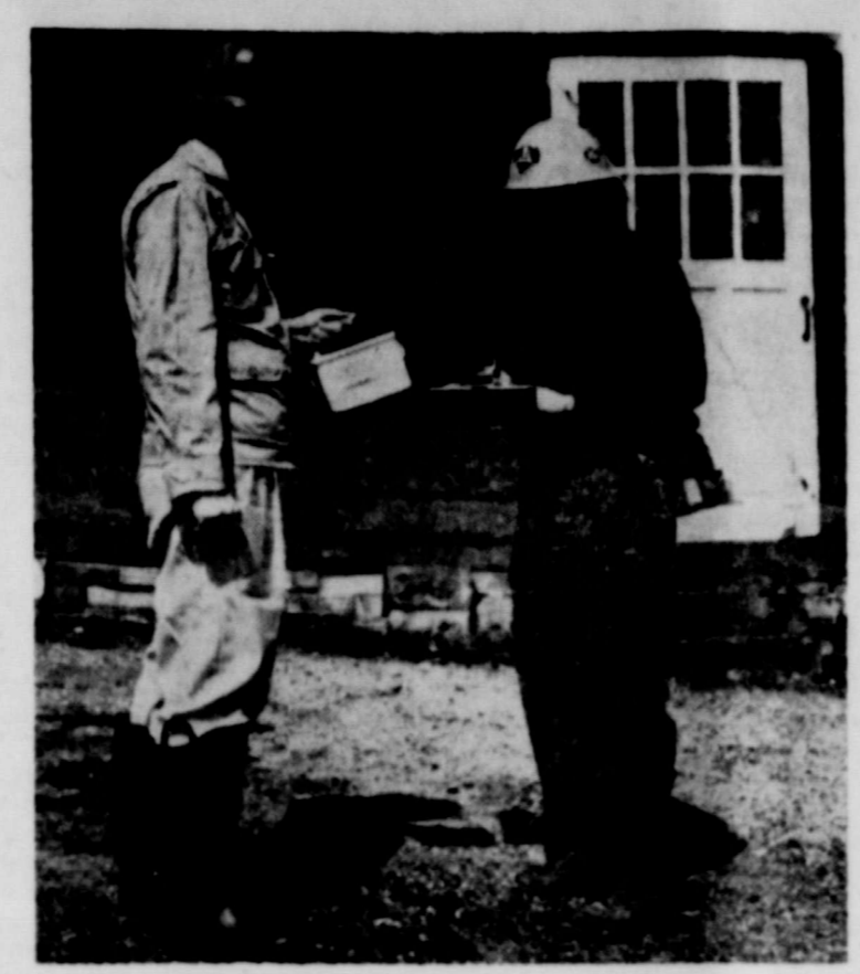
RADIOLOGICAL MONITORING team checks a damaged area for "radioactive fallout" just as would be done after a real nuclear attack. Similar teams also carried out simulated missions in various parts of the nation during the July 8-19 Operation Alert 1957, a nationwide training exercise to strengthen the country's non-military defense against possible attack. The man at left is using a radiological "survey meter," while his partner is recording the intensity of radiation from the simulated fallout. (FCDA Photo)
