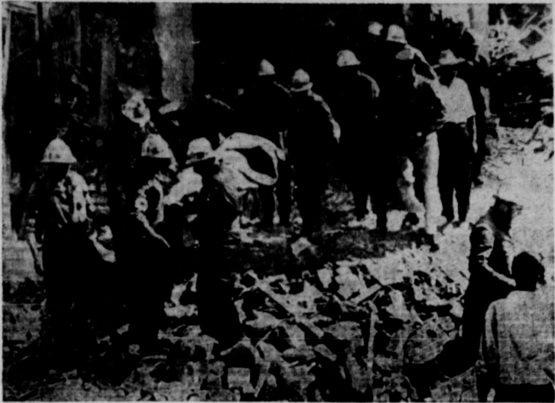
QUAKE WRECKS TOWN . . . Firemen carry body from ruins of Baudoin Hotel in Orleansville, Algiers, where earthquake killed 1,600 and demolished one-fifth of the city, rendering thousands homeless.
