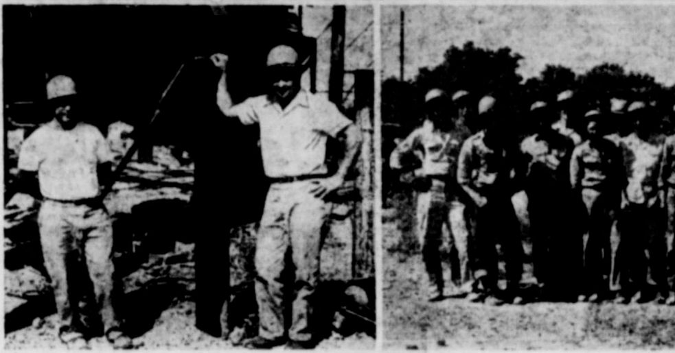
NEW TRANSMISSION LINE ENERGIZED.—Community Public Service Company's new 66,000 volt line from Hamilton to Gatesville, Texas, has been placed in service, completing a 66,000 volt "loop" serving the company's Central Texas properties. At top left is a view of Community's Hamilton County substation, one mile northeast of Hamilton, with new transmission line to Gatesville leaving substation, with facilities for automatically switching the new line. At right, top right shows view of new addition to Hamilton County Lower left, Jake Perry, line foreman in charge of the construction standing before the 66,000 volt oil switch in substation addition. Bottom right is Community's Central Division line crew, which built the line and substation addition. (Photo and story courtesy of CPS Co.)
