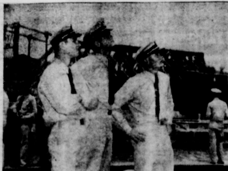
WATCHING OPERATION OF CRANE AT THE PANAMA CANAL are Midshipmen (left to right) John J. McCorkle, Dudley D. McCalla, and Benjamin T. Rhodes Jr. Midshipman Rhodes is the son of Mr. and Mrs. Ben Rhodes of Cranfills Gap. Midshipman McCorkle is from Fort Arthur, and Midshipman McCalla is from Austin. All are students at the University of Texas. They participated in "Cruise Charlie," one of the Navy's three 1953 ROTC Midshipman Cruises to foreign ports. Some 5,500 officers and men including 1,100 Midshipmen from 32 colleges and universities manned the 11-ship training squadron under the command of Rear Admiral Richard P. Glass, USN. Ports of call included Colon, Panama; Port-of-Spain, Trinidad; and Guantanamo Bay, Cuba. The cruise ended August 29. (Official U. S. Navy Photograph).
