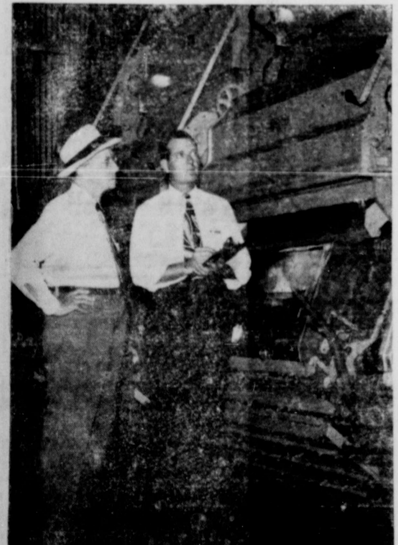
ONE OF TEXAS' hundreds of cotton gins is checked for fire hazards by an inspector (center) for the Fire Prevention and Engineering Bureau of Texas. Bureau inspectors visit more than 2,000 gins, industrial plants, warehouses and other large buildings annually in their never-ending effort to reduce Texas' mounting fire losses. The Bureau, which is owned by the fire insurance companies, makes no charge for its services.
