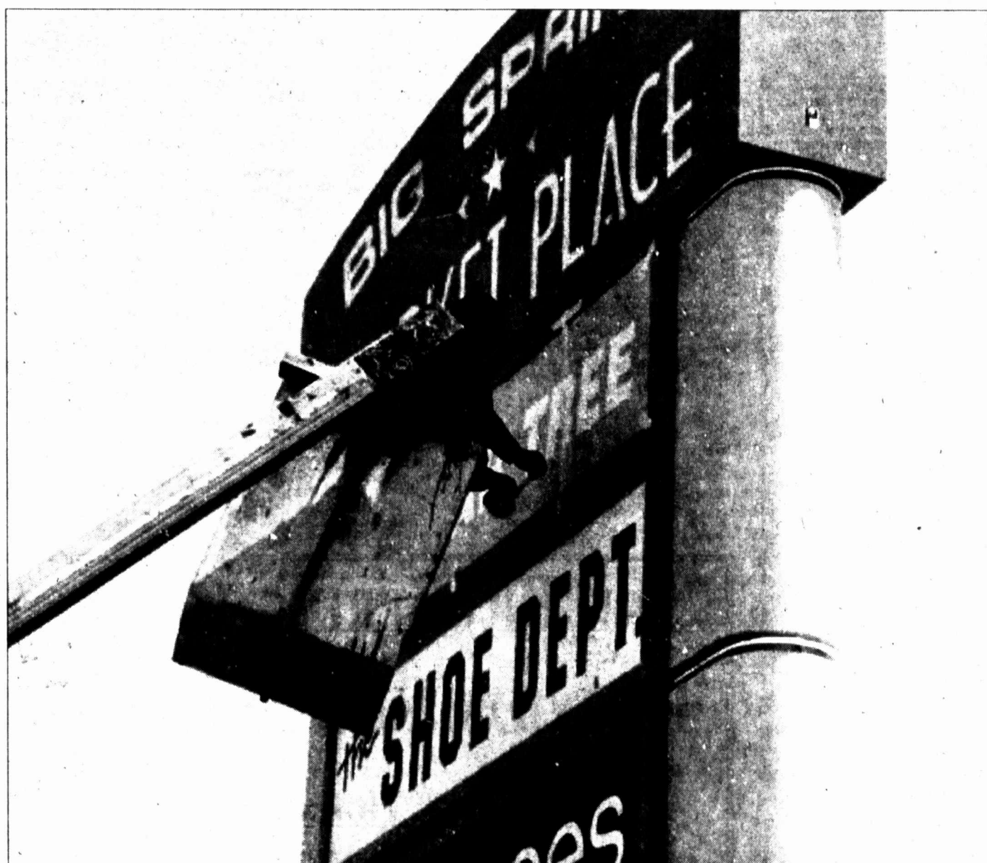
HERALD photo/Thomas Jenkins An employee with Permian Sign Company affixes the Dollar Tree name to a sign at Big Spring Market Place, located adjacent to Wal-Mart. Each day, workers move a little closer to getting Big Spring's newest retail center up and running.
