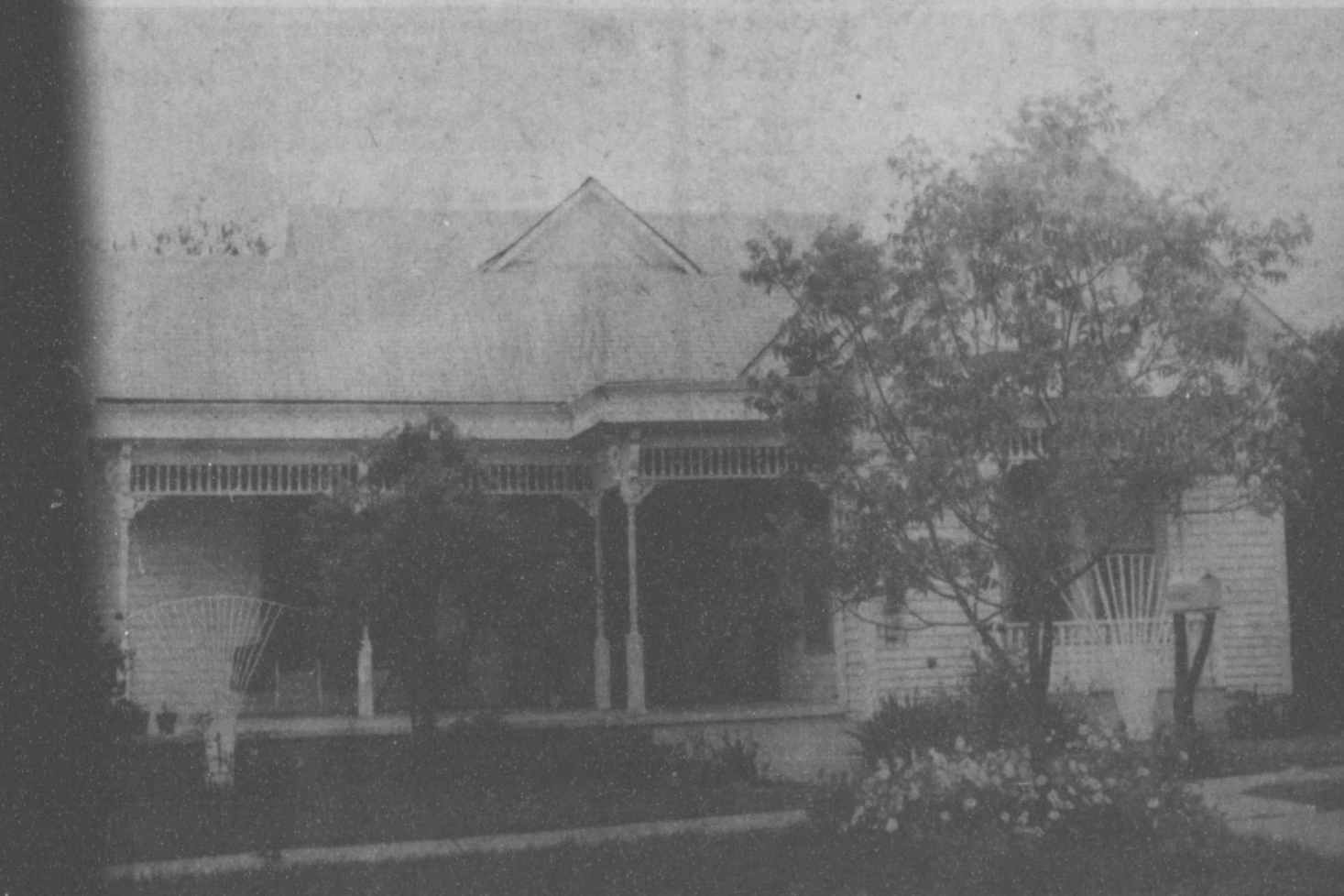
The C. E. Shirrey home located at 406 South Seventh. The house has recently been painted and had some work done, so Mrs. Shirrey was proud of the improve-
