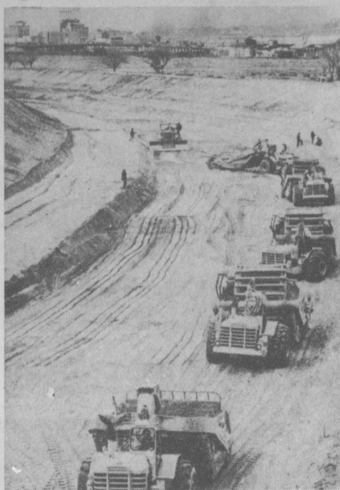
Loaded to the gills and lined up Indian file, this fleet of Allis-Chalmers earthmovers tote away more than 25 tons of sand and dirt from the new river bottom forming the relocated channel of the Rio Grande.
