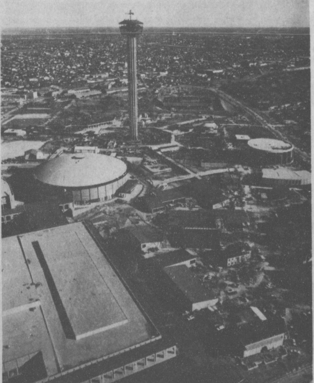
WORLD'S FAIR—HemisFair '68, only a dream a few short years ago, stands proudly in San Antonio as the last month of work continues before the April 6 opening. The $13 million civic center complex in the foreground, 622-foot Tower of the Americas in the center and the $6.75 million United States Pavilion on the right center are all prominent in the picture of the 92.6-acre showcase.
