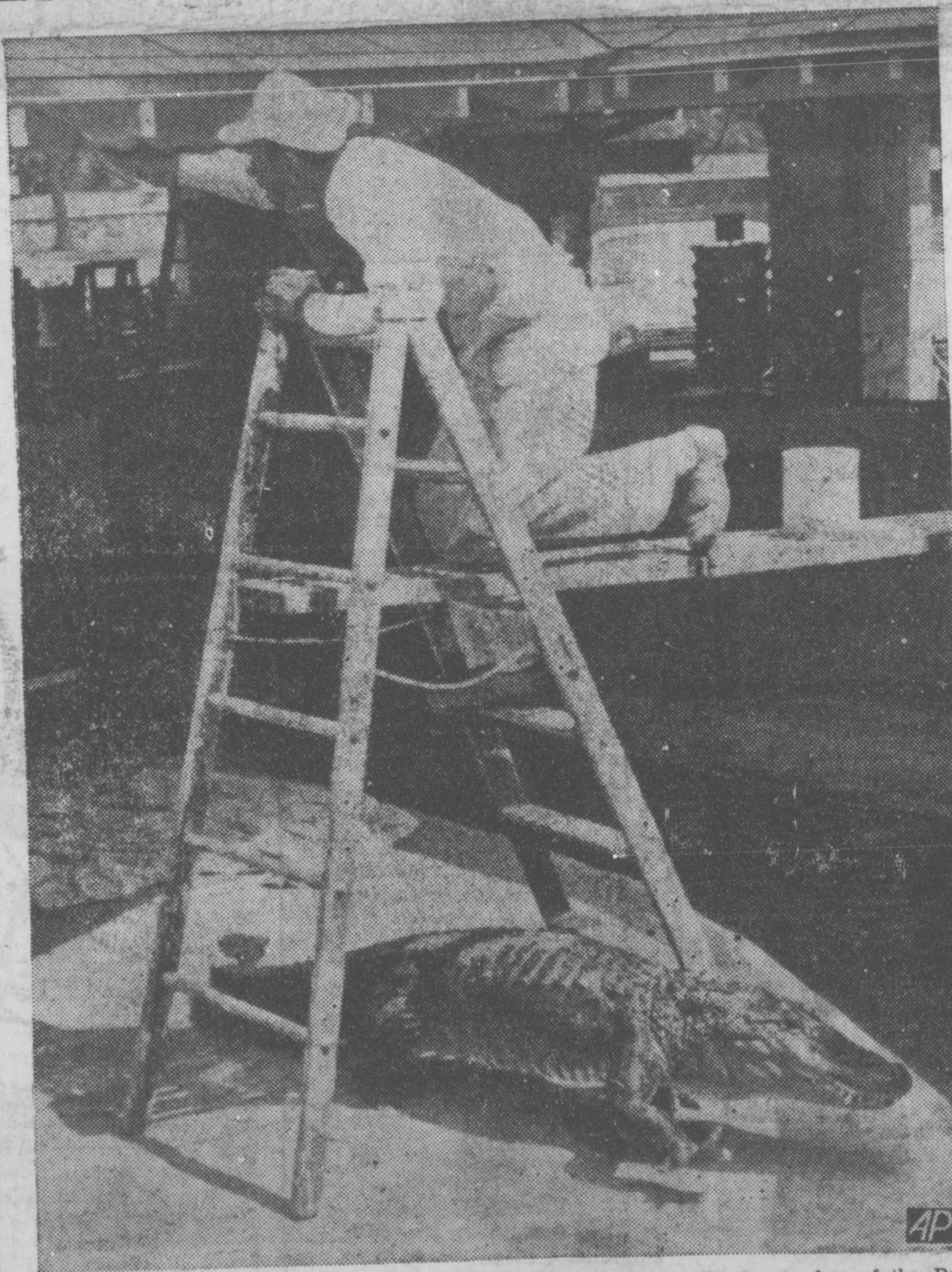
WORK HAZARD — A man just has to ignore the hazards of his job sometimes if he's going to get any work done. And for painter Juan Rivera those hazards are sometimes pretty strange. Rivera displays healthy nerves as he paints the shelter at the alligator gardens of the Breckenridge Zoo in San Antonio.
