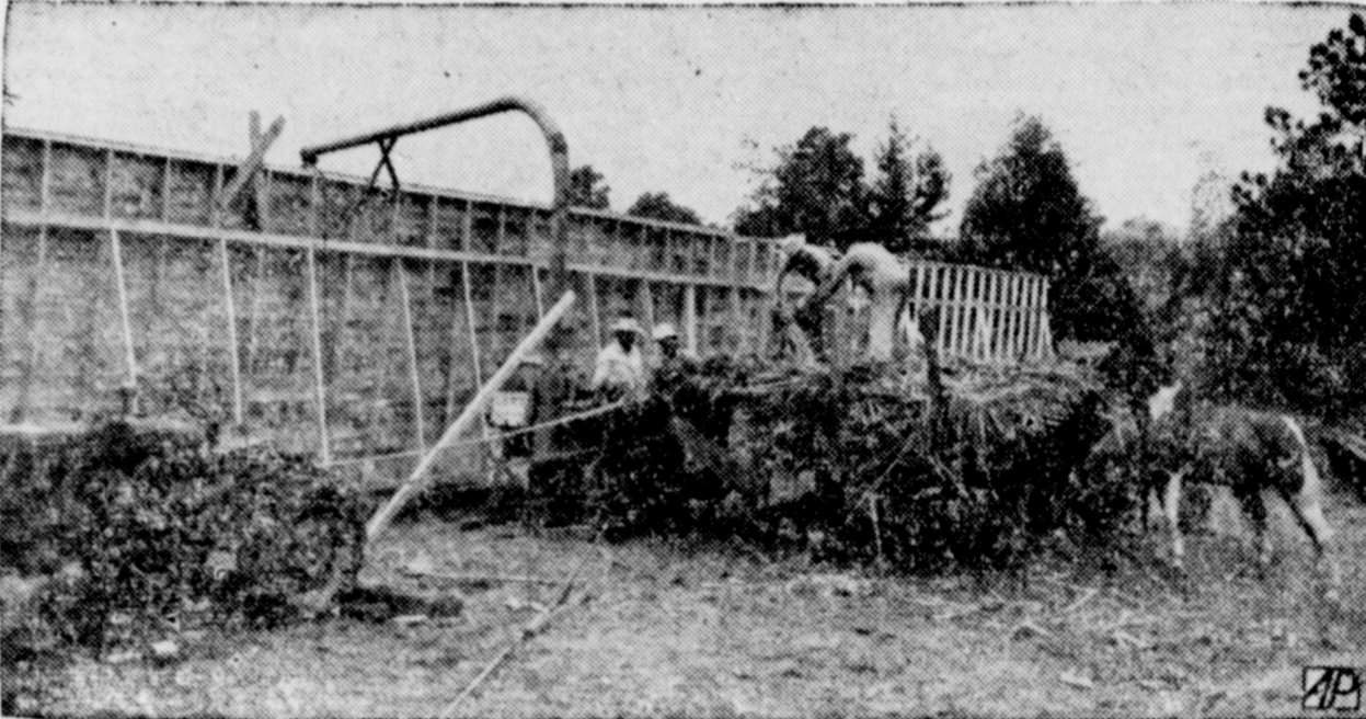
CONSTRUCTS BOX SILO
