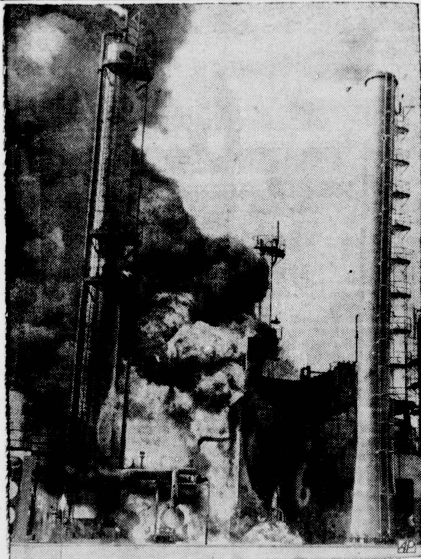
REFINERY FIRE— Flames boil around one unit of the polymerization plant at the Continental refinery plant in Wichita Falls. Refinery Superintendent John A. Ramsey said the fire was caused by a ruptured tube in a re-boiler. Damage was estimated at $5,000 to $10,000.
