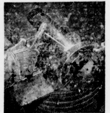
THEY WELD PIPE
