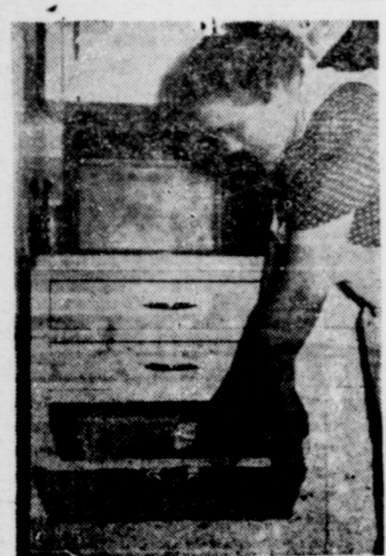
A hopper designed for the lower part of a kitchen cabinet makes wastebasket tending a thing of the past in Mrs. I. E. Meyers' kitchen in Wood County, Ohio, points out nationally-circulated Capper's Farmer. It connects by chute with the basement fuel bin.
