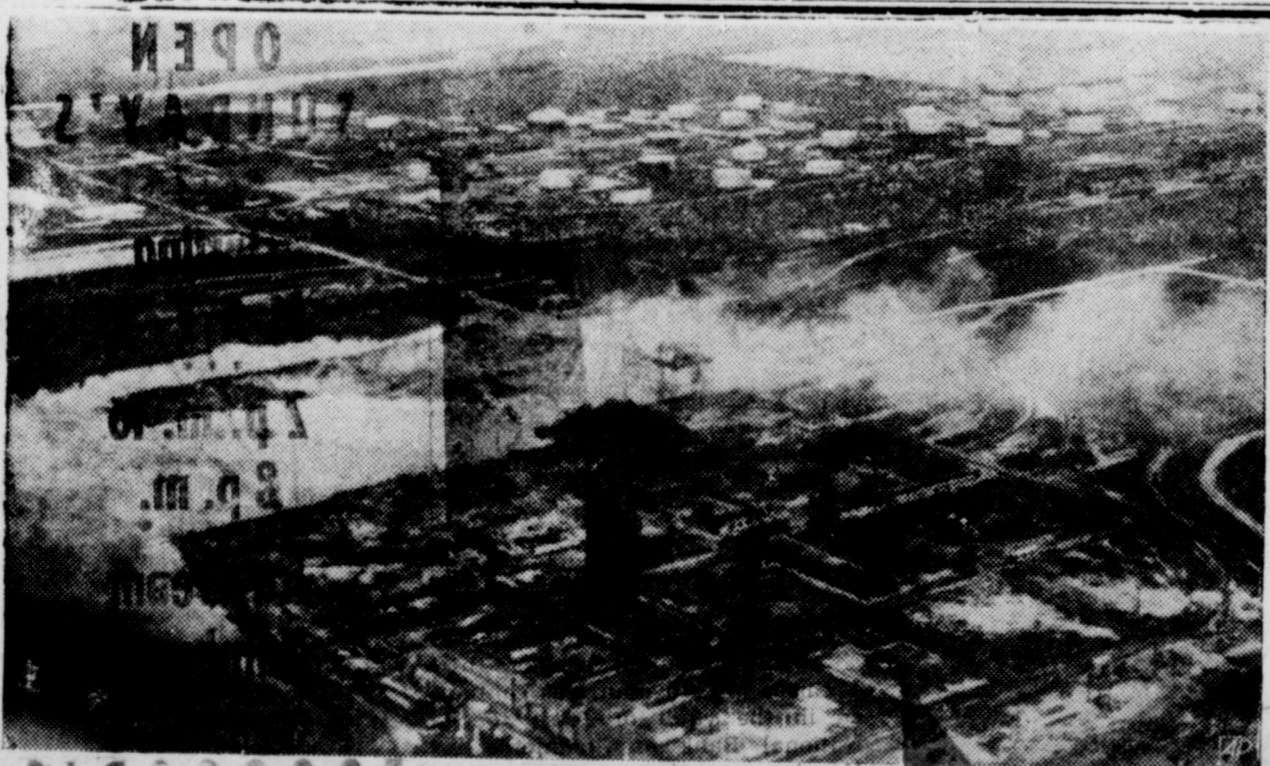
FIFES DIE AWAY IN DISASTER AREA This picture from the air, a ravaged Texas city, shows the devastated area after flames had died to a few smouldering beans. The plant (foreground); the dock area (left), and much of the tank farms
