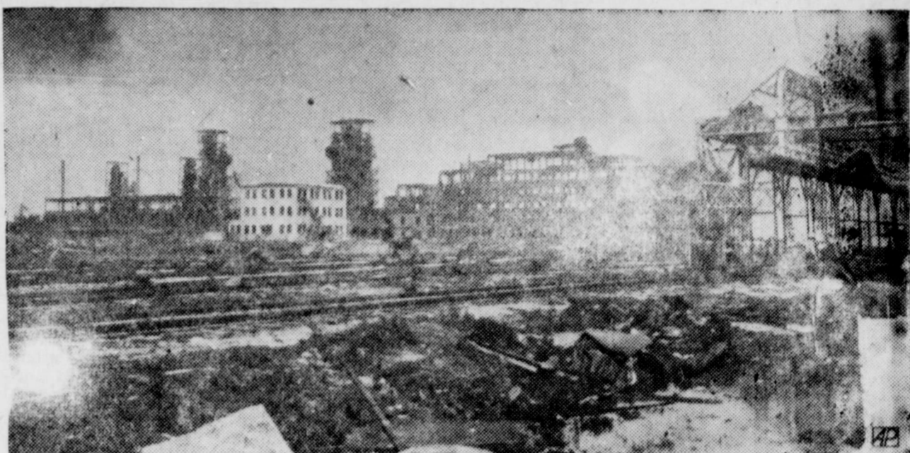
DESOLATION AFTER BLAST! as City on April 21, five days after explosions and fires which will be rebuilt on the same site. This desolation, reminiscent of the ravaged much of the Texas coast- (AP) Wirephoto. Monsanto Chemical plant to Texas community. Company officials
