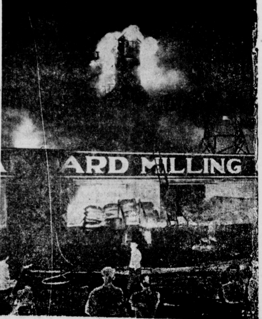
Flames spurt from an elevator of the Standard Milling Company at Lubbock, Texas, just before an explosion ripped off the sides. The fire raged for four hours through warehouses and grain-filled elevators of the company. (AP wirephoto).
