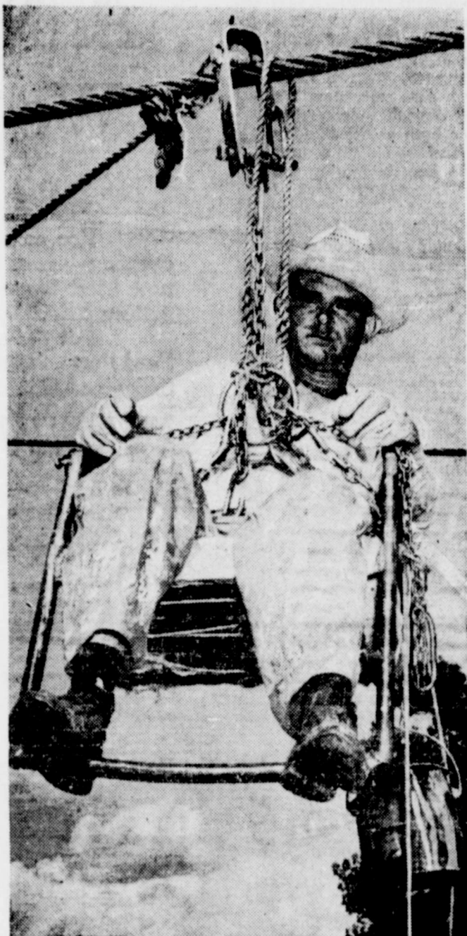
Invented by members of Lone Star Gas paint crew this boatswain's chair enables them to paint pipeline suspension bridge rods in less time than they used to require. It was designed primarily for the safety of the painter.
