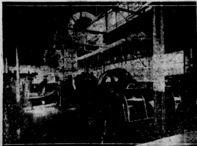
The huge power plant at the sugar company's mill at Clewiston.
