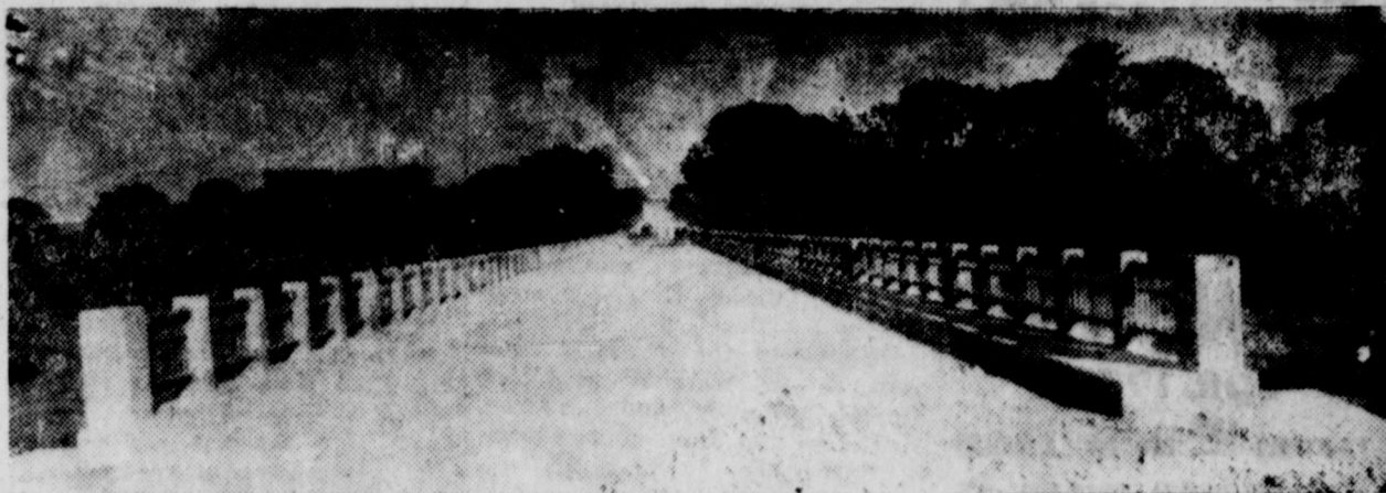
Looking east across new Leon River bridge, Highway 7, at Gatesville. Photo taken by Mayes at completion of bridge before approaches were finished. Engraving cut made by the Coryell County News.
