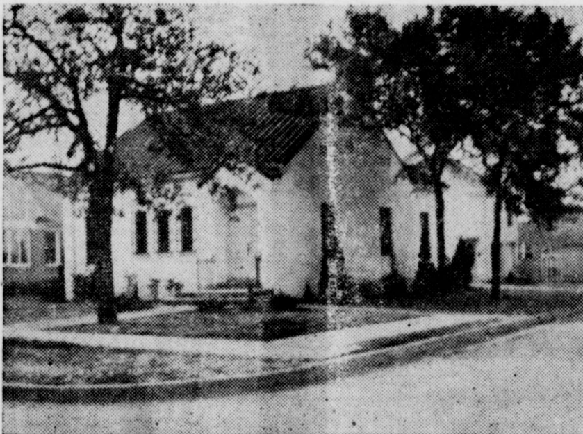
The new Gulf States Telephone Company building, which has just been completed and was occupied ten days ago by that company. After everything has been completed the company intends to hold open-house, inviting the general public to view the new building and see the new plant in operation.
