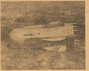
A 150-pound, 5½-foot "Grasshopper", resembling a small homb, is going to the Antarctic on "Operation Deepfreeze" during the In-ternational Geophysical Year 1957-58. The Navy intends to use the super-robots as weather relay stations after parachuting them to desired locations. (FHTNC)
