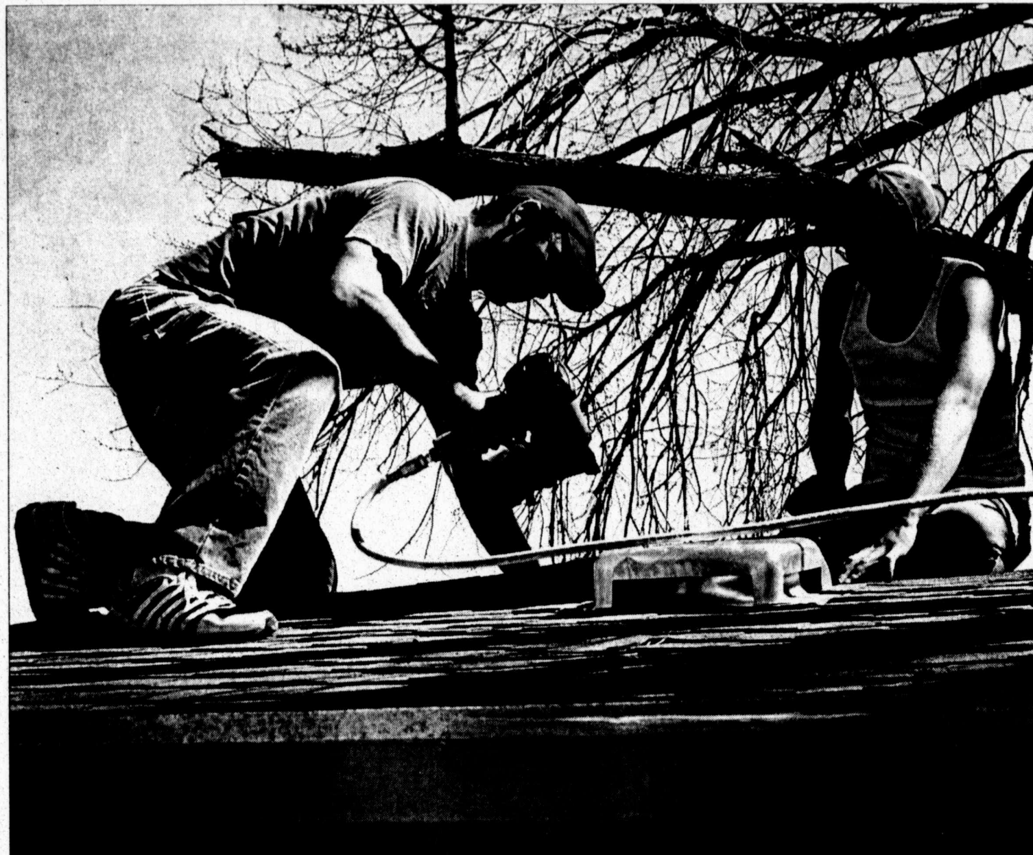
HERALD photo/Steve Reagan Big Spring High School Construction Technology students Talbott Moore, left, and Joe Richter work on roofing a shed at the high school Friday afternoon. The building-trades program at BSHS was recently re-started after being dormant for more than a decade.
