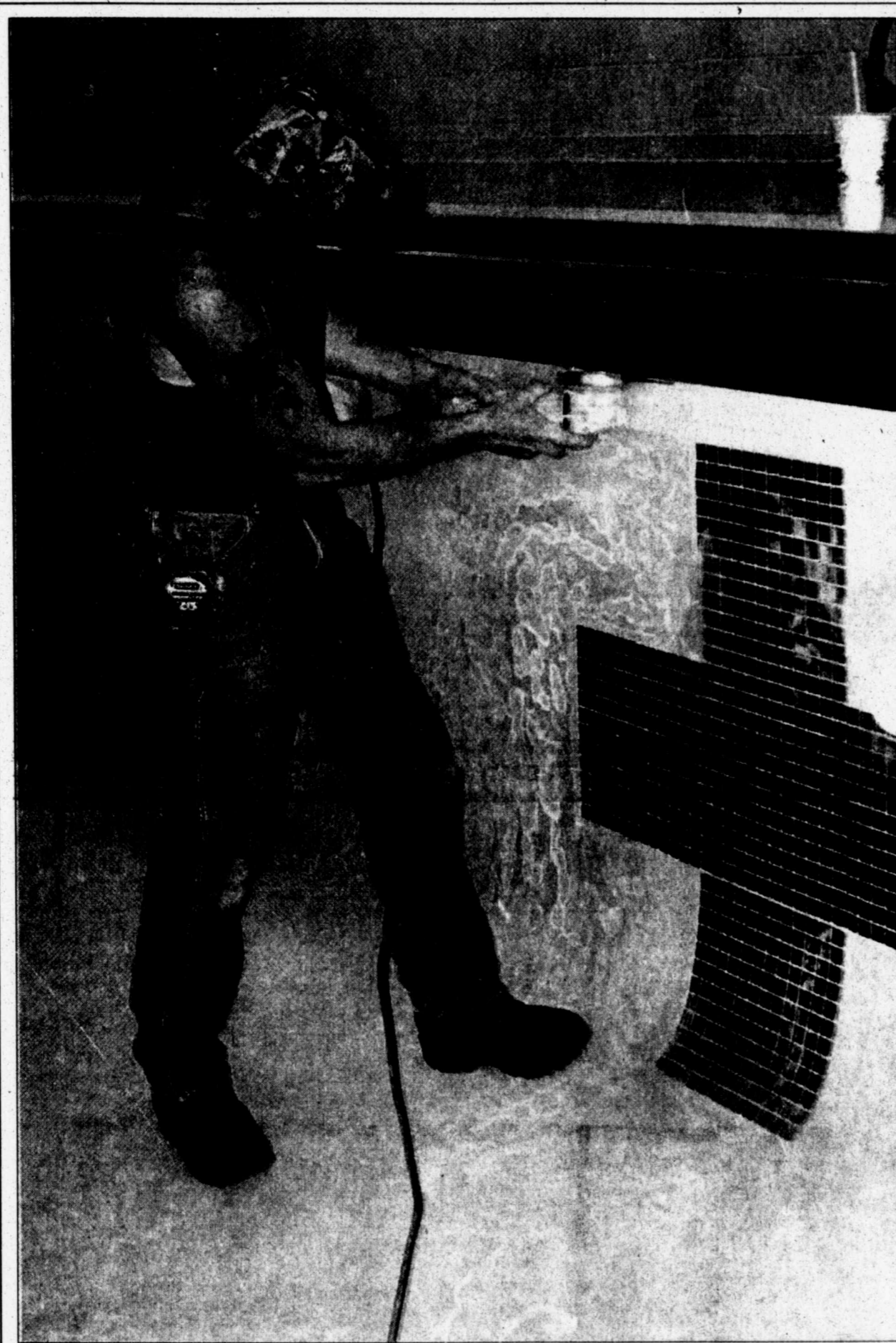
John McGhee, an employee of Renosys Systems, uses a grinder to cut notches into the side of the swimming pool at the Big Spring YMCA. The notches will be anchor points for a new vinyl lining for the pool.
