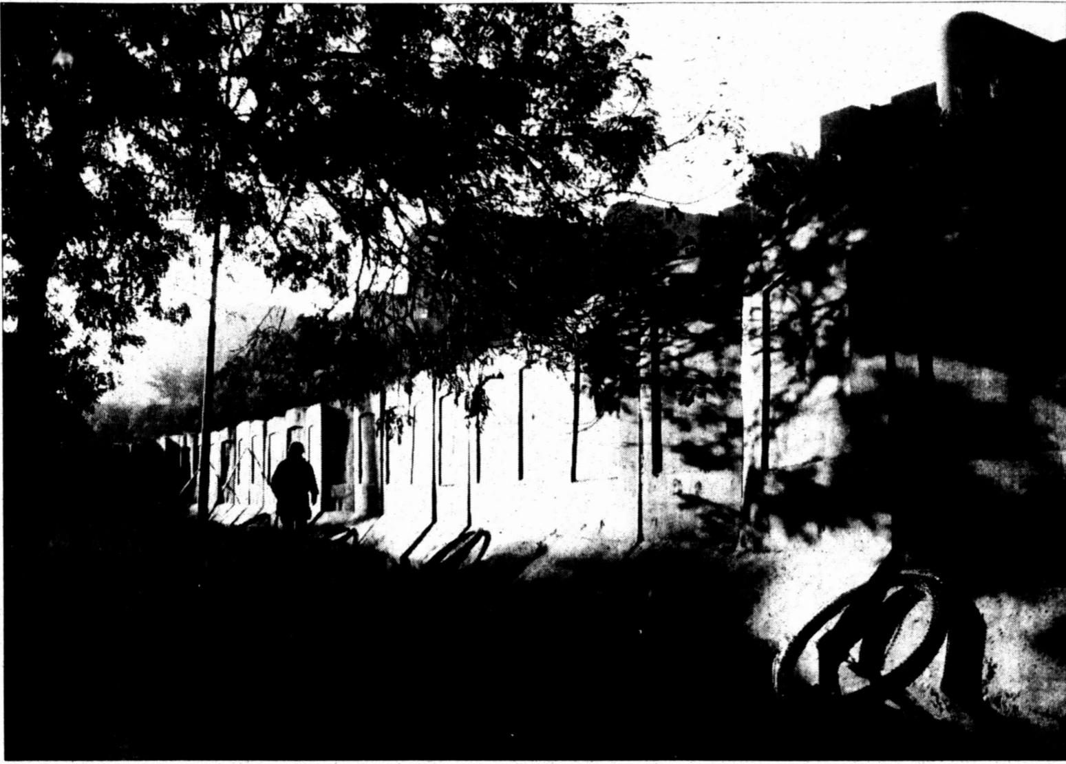
U.S. combat engineers constructed this concrete blast wall on Haifa Street in Baghdad, Iraq, to provide protection for a palace occupied by U.S. forces.
