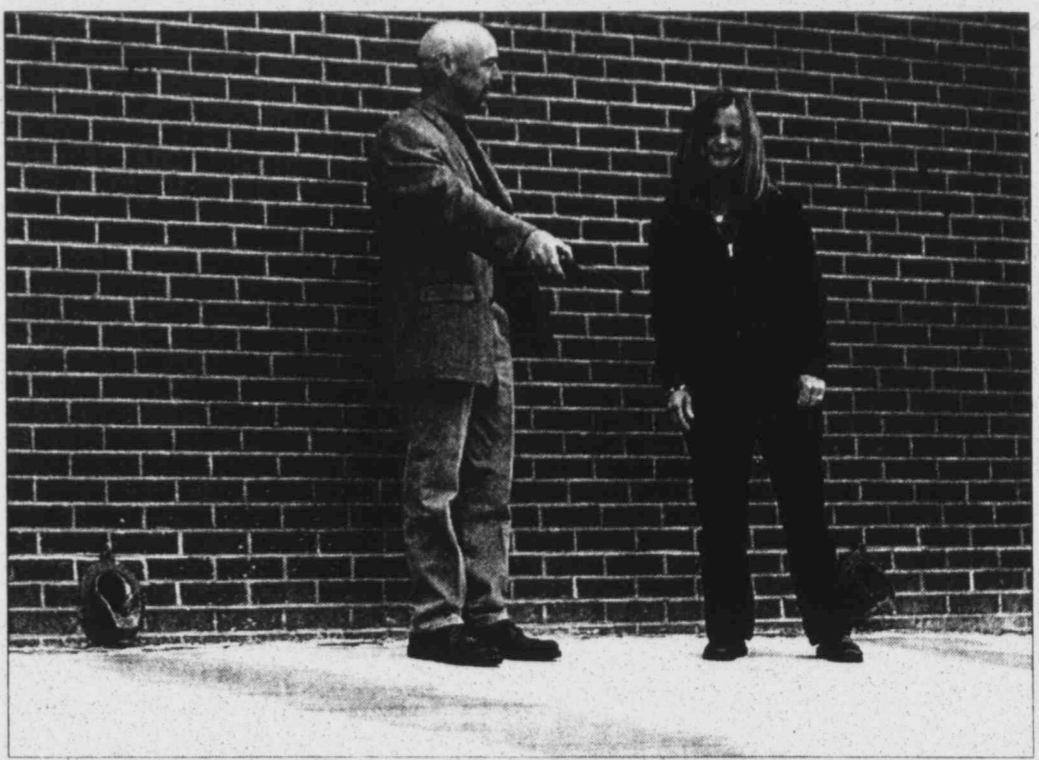
HERALD photo/Kendra Wiss Big Spring Junior High School Principal Coby Norman and Grades Clerk Patricia Shanks check to see that the water is being adequately drained away from the building's foundation. The concrete project was completed last week.
