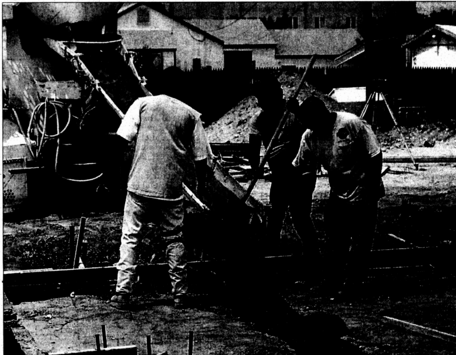
Design Services employees Donnie Hernandez, right, Enrique Enriquez and Pancho Huerta lay concrete at a lot on Gregg Street. The Midland-based construction company is in the process of building a new car wash at the location, which is next to Kwik Kar Tune and Lube.
