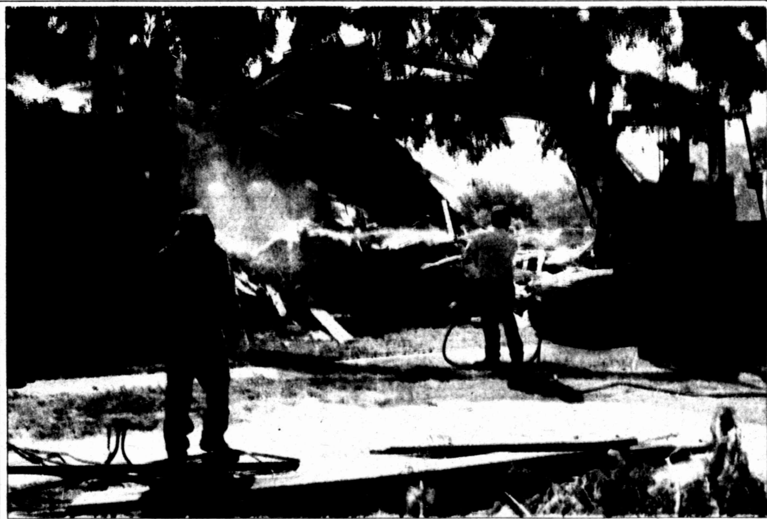
HERALD photo/Lyndel Moody Earthco employees Jesse Salazar, left, and Charlie Martinez assist Johnny Flores who is using an excavator to tear down the old Howard Cottage building. Workers had the structure torn down in a matter of hours Wednesday and are continuing to haul off the debris. Removing the old Air Force barracks now paves the way for the college to move ahead on a multi-million dollar visual and performing arts center.
