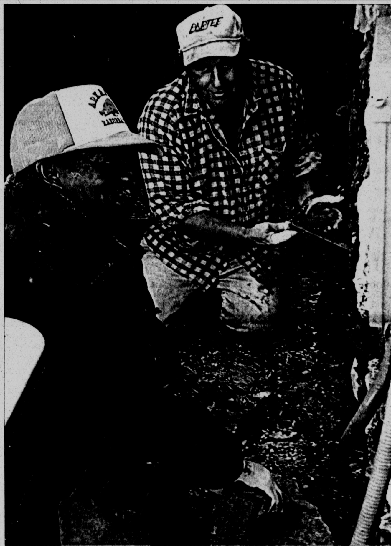
Riley Falkner, right, and Thomas Lewis of Falkner Masonry, repair rock work on the exterior of the House of Hope building on Scurry Street. Work continues to progress on the building's remodeling project through volunteer efforts. Birthright, an independent organization dedicated to providing resources to pregnant teen-agers, moved into the south portion of the building this week.
