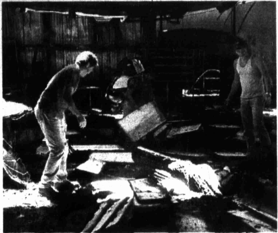
HERALD photo Employees of Solitaire Homes sift through the wreckage of a fire that ripped through the manufactured home plant in May of 2002, causing more than $1.5 million in damages. The plant is expected to re-enter production by the end of the year, according to Moore Development for Big Spring Inc. officials.
